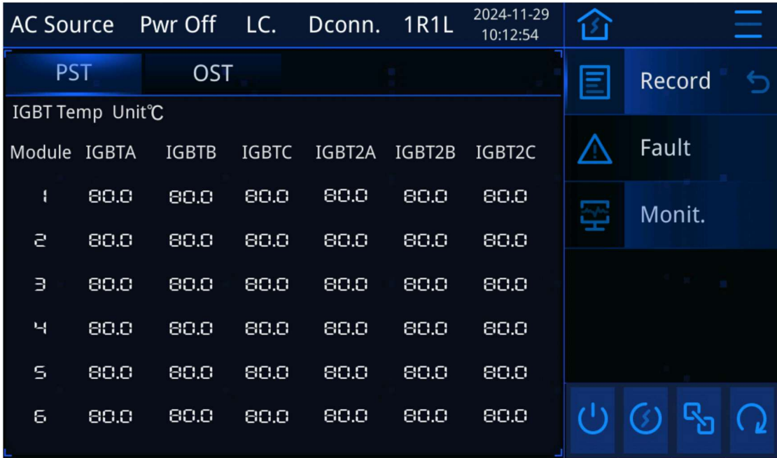
Figure 5-66: Front-stage Temperature Interface
