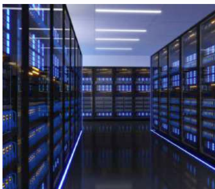
Server Power Supply Reliability Testing
